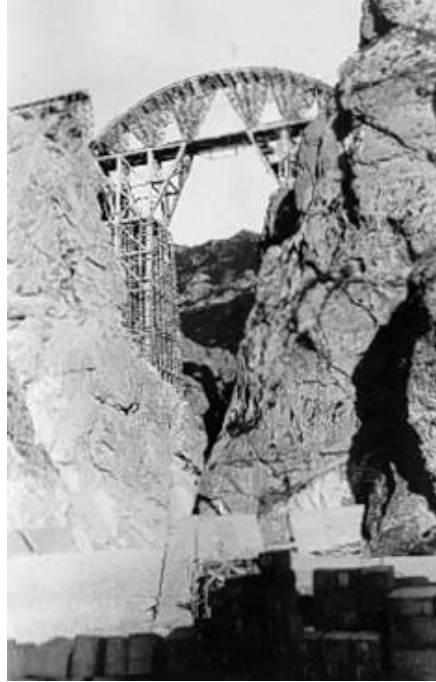
Photo 25: The completion of curved slab forming
