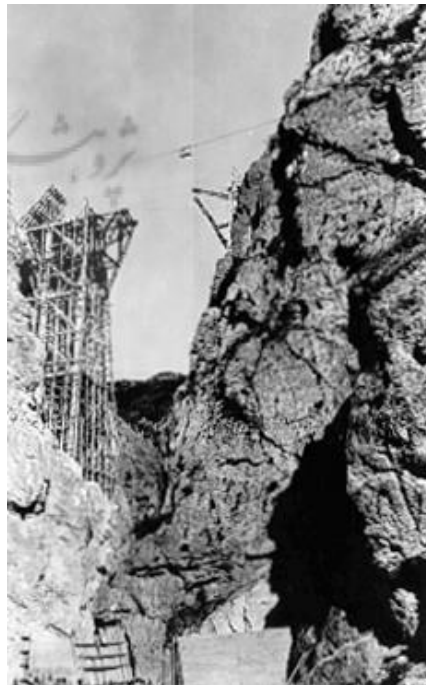
Photo 18: Transferring of materials and precasted elements using the cable.
