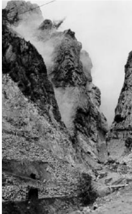
Photo 1: Explosion operation is conducted to provide enough space to install falsework. The cable which is connected to each side of the valley used to transfer materials is shown.
