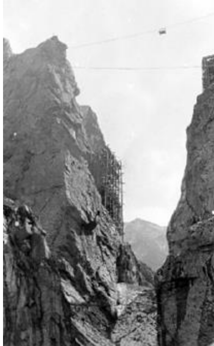
Photo 5: Development of construction operation for the falsework. The concrete structure is built in the falsework.
