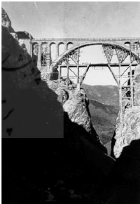
Photo 34: Construction of the brick bridge
