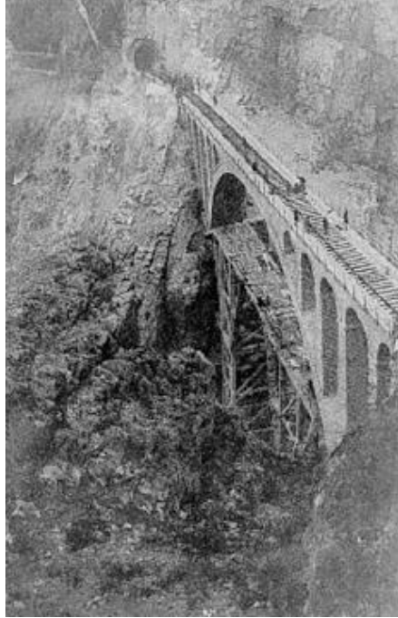
Photo 41: Installing ties and rails
