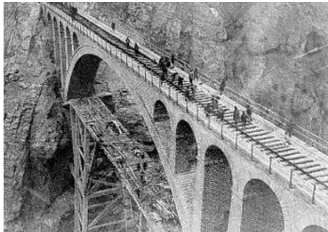
Photo 40: Installing ties and rails
