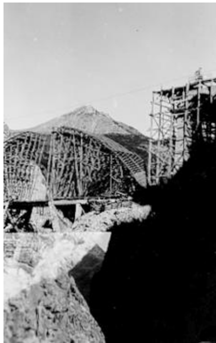
Photo 24: A view of two parts of curved slab and opening and ending of the tunnel
